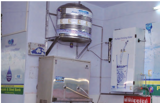
Figure 6: Installation of Trunz Wall Mounted (TWM 001)
