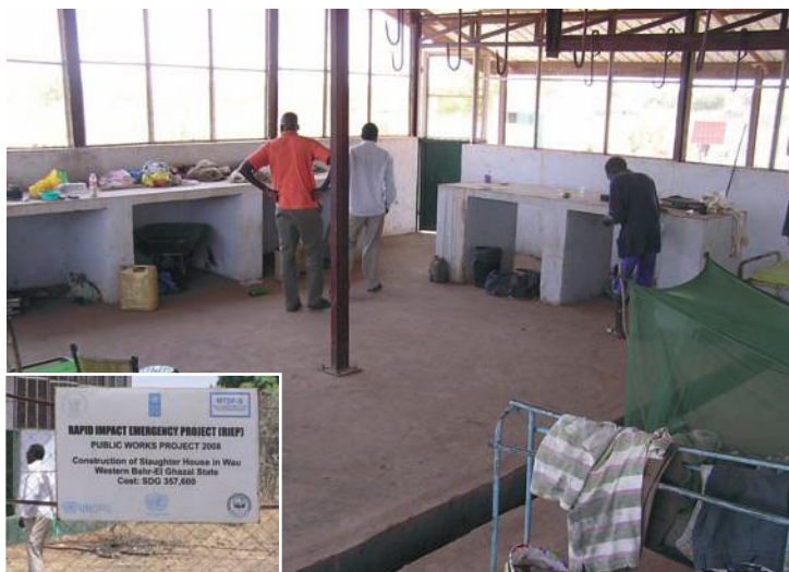
Too many 'white elephants' litter the landscape of the developing world – at least this unused 'improved' slaughterhouse provides a home for two families
